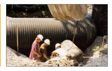
long pipe joints were aligned using flexible creosote resistant, nitril couplings prior to extrusion welding of the inside joint surface. Each joint was successfully air tested to 5 psi prior to E.P.A. approval.
